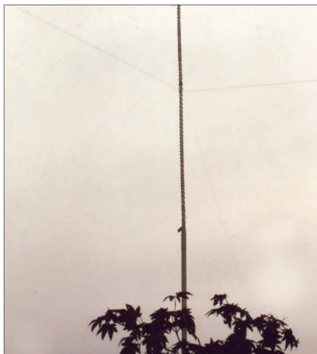
Fig. 4: Jonathan Kempster M5AEO’s low profile antenna is about 4m (13 feet) tall, which is almost invisible from the ground as it’s mounted around 18m above ground.
