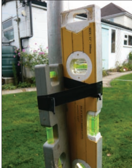
Two spirits levels to make sure the support pole is truly vertical when it's embedded in the ground.
