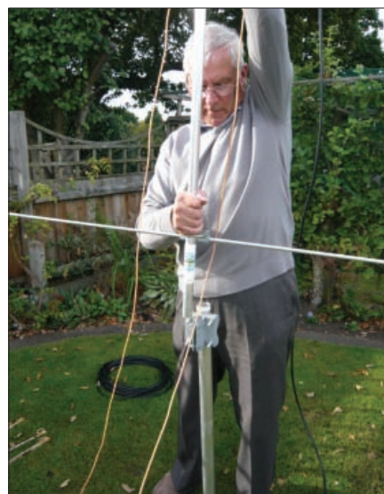
Dave G3ZPR, lifting the completed antenna up onto the supporting ground post.
